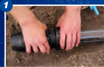
1 Use the multi-grips to loosen the nut then continue to loosen by hand and slide the body off the pipe.
