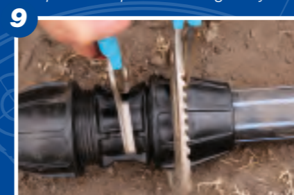
9 The fitting is now fully installed
