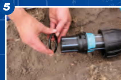
5 Slide the components onto the pipe, first the nut, then the split ring and collet followed by the O-ring.
