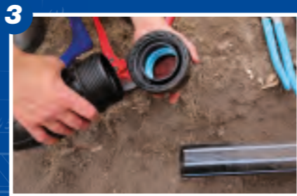
3 Take the fitting apart, remove the nut.
