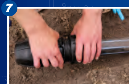
7 Tighten the nut by hand.
