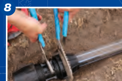
8 While holding the body tighten the nut all the way to the flange using multi-grips
