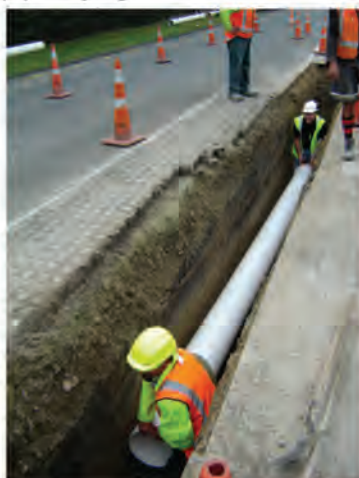
Figure 7.1 – Potable water pipeline is easily manoeuvred in the trench during installation.
