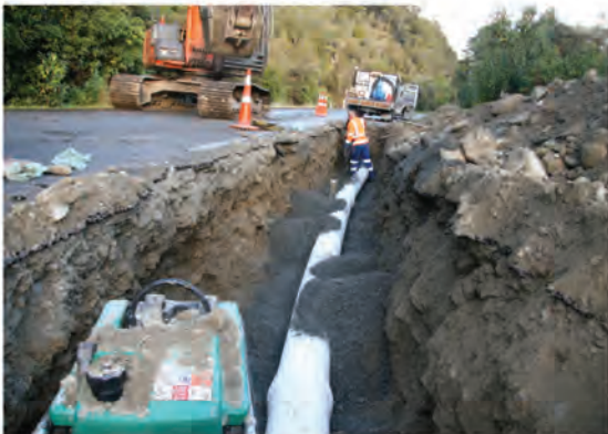
Figure 7.6 – PVC-U curved pipeline following road curvature.
