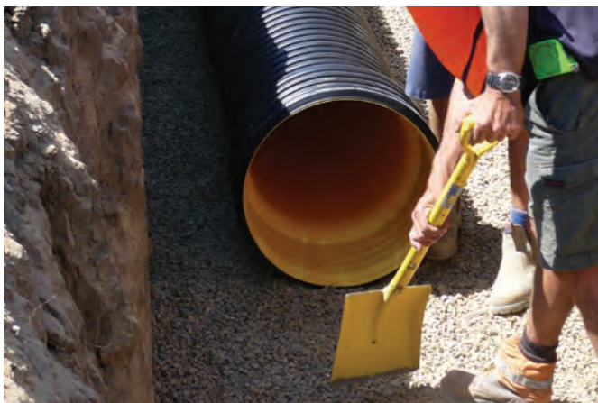
Granular material spread evenly in the trench
