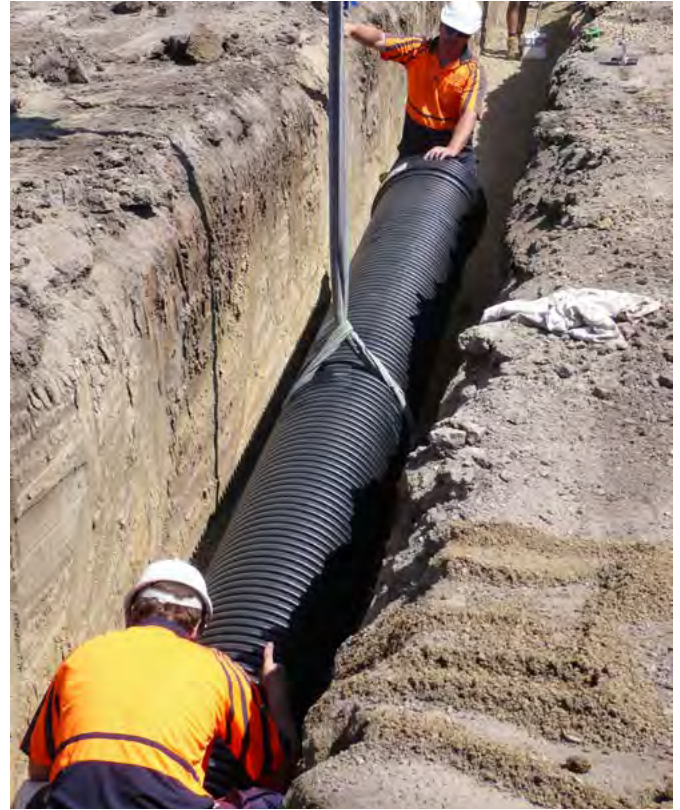
BlackMAX® pipes lowered into the trench with a nylon sling
