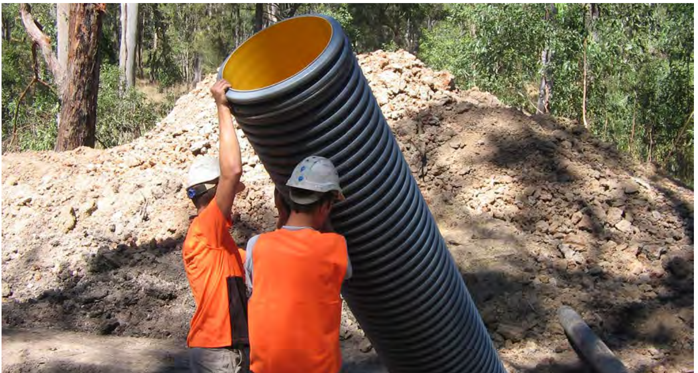
DN600 SewerMAX® pipes in 3m lengths are easily lowered in deep trenching
