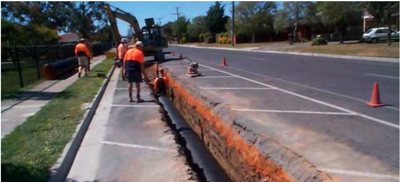
DN600 BlackMAX® stormwater drainage pipes installed under roadway
