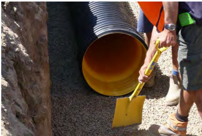
Granular material spread evenly in the trench
