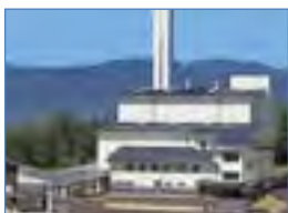
15 Waste incineration plant
