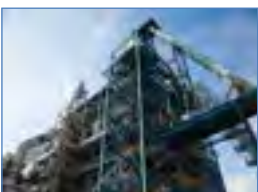
16 Biogas power generation plant
