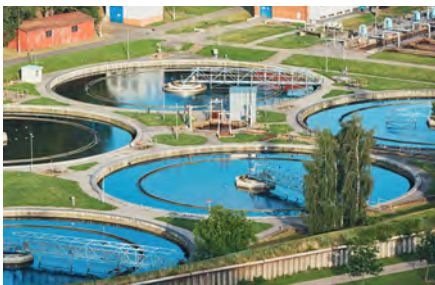
Water / Wastewater Treatment
